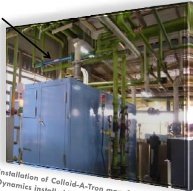
Installation of Colloid-A-Tron manufactured by Fluid Dynamics installed in the supply of water cooling the compressor
