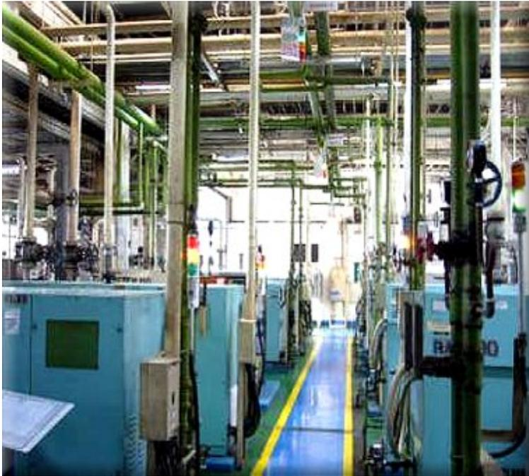
A series of 220 KW air compressors and air dryers generating compressed air which is used to power various equipment throughout the plant.
