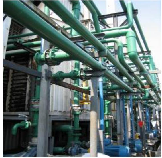
**B-2** Water pump 22 Kw , 30 HP , pipe diameter is 4 inches.
