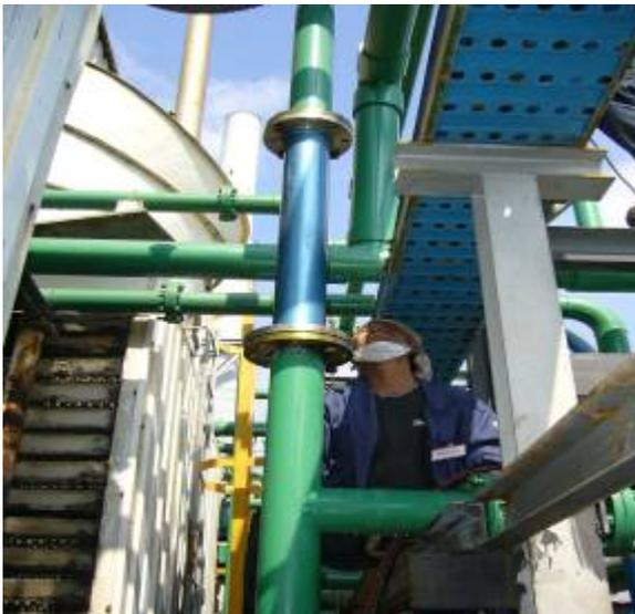
**B-5** Install CAT-100 with flange-ANSI and having bursting pressure 7,900 psi
