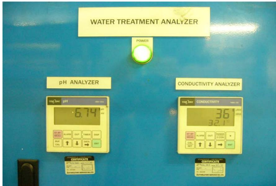
Further to an above data of analyzer , cool water have been proofing a good qualities however there are having a deposit scaling inside pipe and heat exchanger. The mechanism of these factors are
