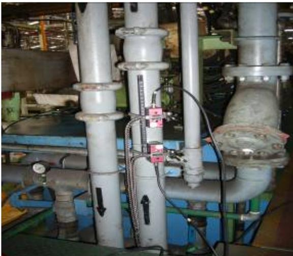
**A-3** Flow Meter installed on the cool water inlet
